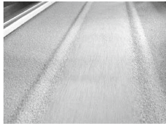
Fig. 3 Photograph shows steady levées with slight slope curvature
